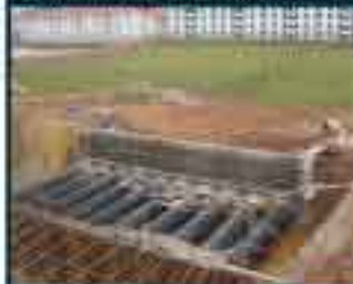
FLOLINE 3-W HDPE PIPES FOR STORMWATER RETENTION SYSTEM
