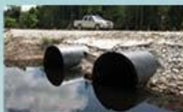
Road Culverts at Jalan Jg. Peking-Tinjar, Baram, Miri
