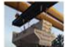
SURE C84 Highway Project 3-Segment Precast Crosshead
