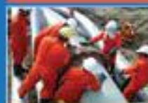
Civil and Mechanical Site Preparation Works
