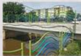
T Beam Bridge
