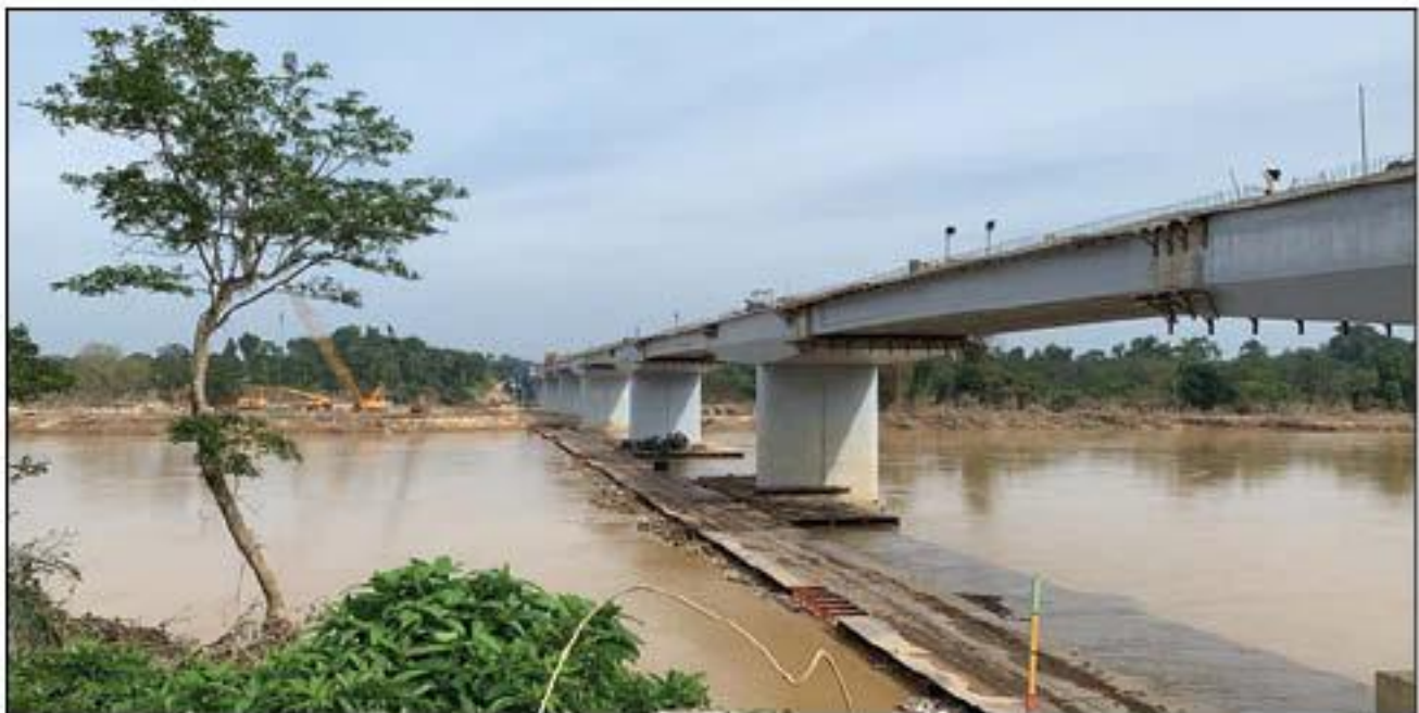
BERA BRIDGE - PAHANG
