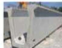
Sunway Link Precast Pre-Tensioned U-1800 Beams
