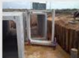
Giant Size Box Culvert
